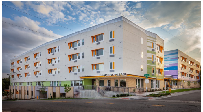
Exterior view facing west, showing the workforce housing entrance.
