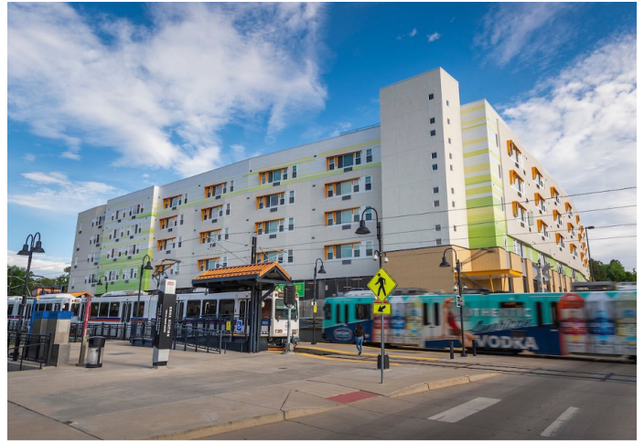
View of Arroyo Village from the Knox Court Light Rail Station.
