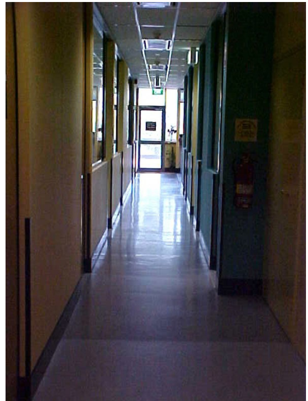
Highly polished surfaces can create reflective glare that creates a difficult visual field for older adults. (HomeFAST: Home falls and accidents screening tools. https://stopfallsathome.com.au/risks/ )
