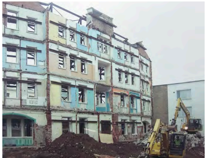
The 2010 renovation of the building removed all but the historic front facade.
